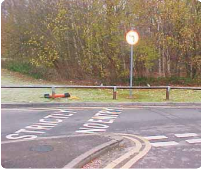
St Peters Hospital - Line Marking and new sign
