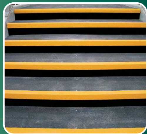
After Covering the galvanised steel
